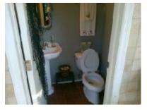
CONDITION OF SINK: Single sink is functioning as intended. Appears serviceable. CONDITION OF TOILET: Appears serviceable. BATH VENTILATION: None or inadequate ventilation noted.
