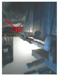
**SECONDARY DRAIN PAN:** On the PVC overflow line, there is a shut off float switch which appears serviceable.
