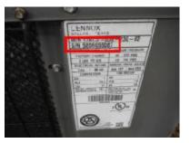
CAPACITY OF UNIT: 3 ton unit. POWER SOURCE: Electrical disconnect present.
