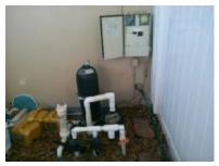
PUMP/MOTOR CONDITION: Appears serviceable. LEAKAGE? No. LEAF BASKET: Appears serviceable. PRIMARY FILTERING: Cartridge, Appears serviceable. PRESSURE IN PSI: 8 psi.
