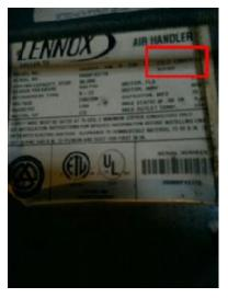
CAPACITY PRIMARY UNIT: The unit is forced air heat strip: 4 KW. CONDITION OF AIR HANDLER: Unit is in fair condition for its age and appears to have been maintained with regular maintenance.
